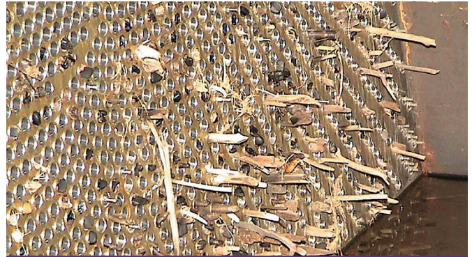
Condenser tubes without debris filter
