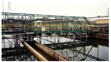
Duffin Creek, ONT– Primary Clarifier Traveling Bridges (77-ft wide x 210-ft long) with cross collectors. Bridge drives are dual independent synchronized.
