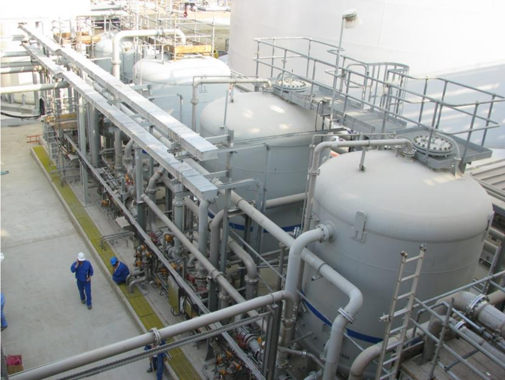
Ovivo Weak & Strong base Anion units with mixed bed Units in foreground
