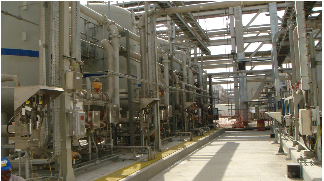
Ovivo Strong acid cation units with mixed bed Units in background
