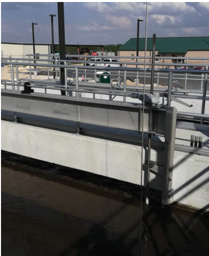
Energy Optimizer®- Automated Effluent Weir Gate
