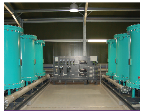
316 m³/h (1400 gpm) Advanced NITRASEP® Plant
