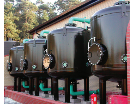
800 m³/h (3500 gpm) NITRASEP® Plant
