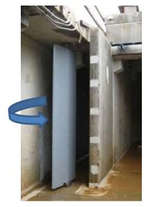
Placed at the entry to the internal recycle (IR) channel, the Eliminat*IR* gate replaces expensive IR pumps and older manual gates. Either the center pivot or the end pivot (common for manual IR gates currently installed) designs are available.
