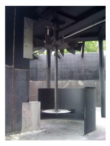
The Excell®Aerator, located at one or more of the channel turns in the Carrousel® Basin, uses the most efficient aerating surface impeller available. The clean water oxygen transfer efficiency is 3.8 lb O<sub>2</sub>/ HP-hr. DHV, B.V., the inventor of Carrousel Systems and the singular authority for testing and certifying Carrousel® aerators has approved the Excell®Aerator.
