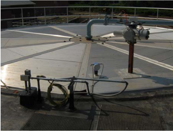
Airbeam Cover Aerobic Digestion System
