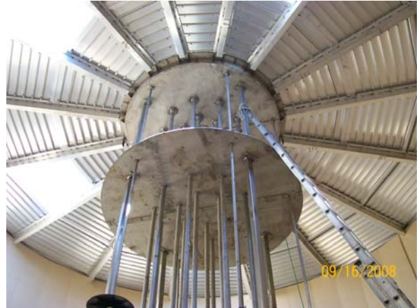
MEDT Aeration Equipment Under the Airbeam® Cover
