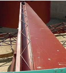
This mechanism covers the entire annular space between feedwell and scum baffles and can eliminate scum quickly and effectively, at a rate faster that that of the standard scum box and skimmer design. This innovative design incorporates a radial approach ramp and an automatic flush valve. The (FTS) is an effective device that will enhance the overall performance of any clarifier of 110' in diameter or smaller.
