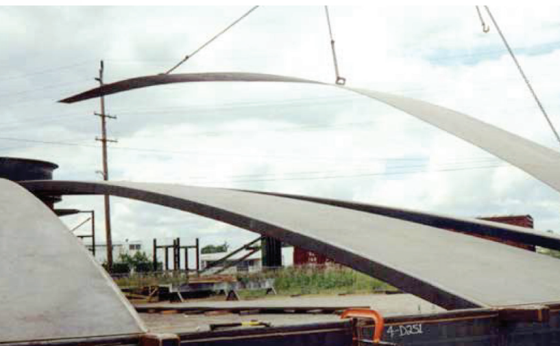
1 Center Ring and Erection Beam Installation
