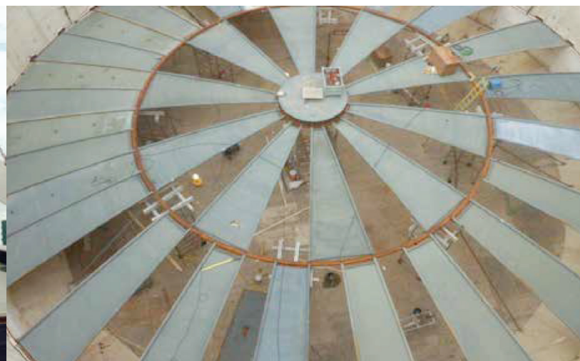
3 Remaining Cover Plate Installation
