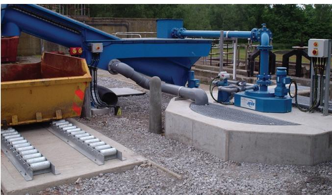
Complete Jeta grit removal systems can be supplied in steel fabricated tanks. These are ideal for attachment to existing flow channels. Jeta® grit trap sizes up to the 550 size can be supplied in this form.
